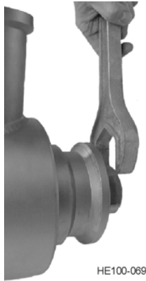
Figure 37 - Installation of Shaft Lock-nut
